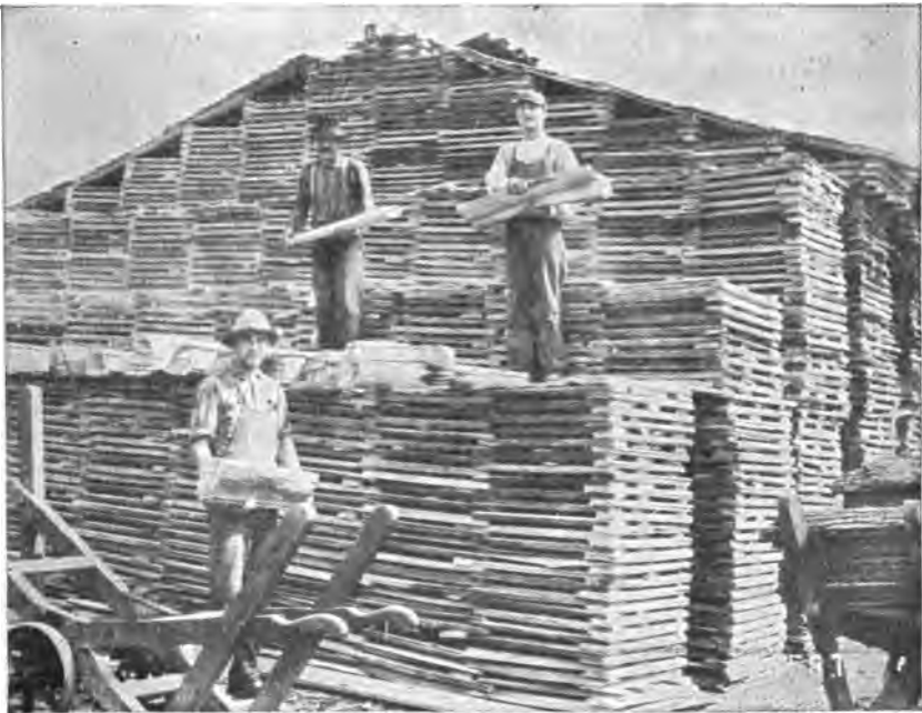
Fig. 22. Piling staves in Ohio.
